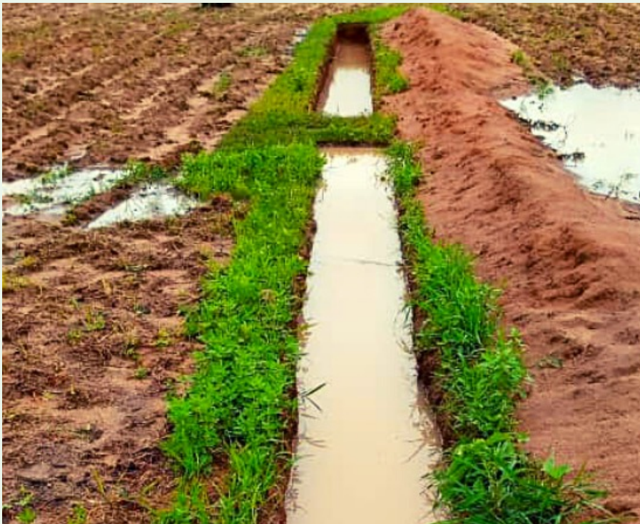
Figure 3 Fanya trench after rains
